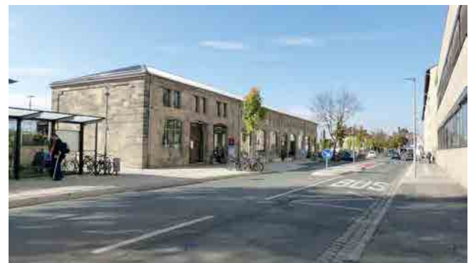
Fahrradparkhaus Brennerstraße Bicycle parking garage on Brennerstrasse
